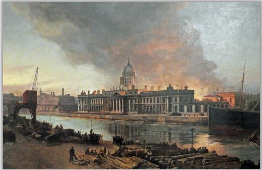
Custom House on fire (Dublin Port Archive)
